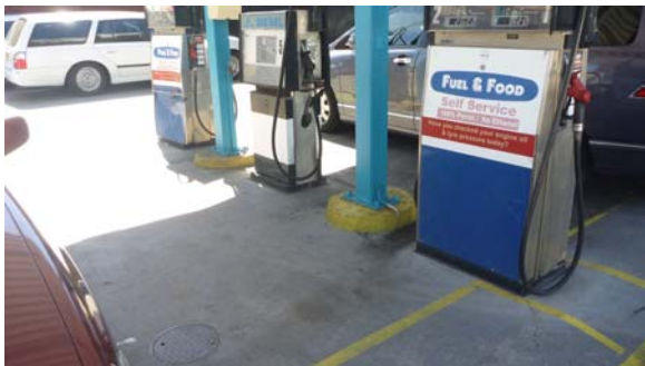
Photo 3: Bowsers at former service station at 650-658 Canterbury Rd, (looking south-east)
