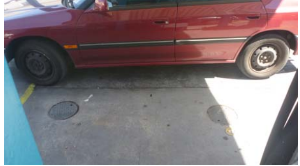
Photo 2: UST filling points at former service station at 650-658 Canterbury Rd, (looking north-west)
