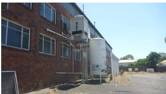
Photo 10: AST area attached to outer central-south factory wall at 2B, 2C-2D Liberty St (looking north-east)
